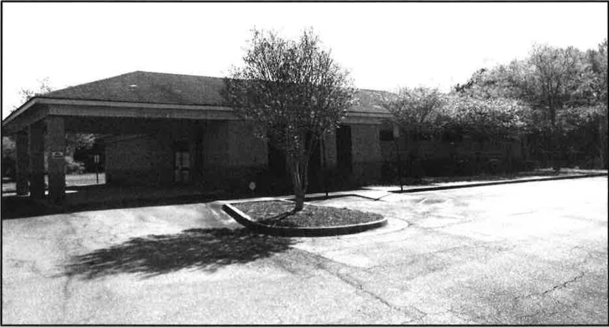
Front View of Subject Building
