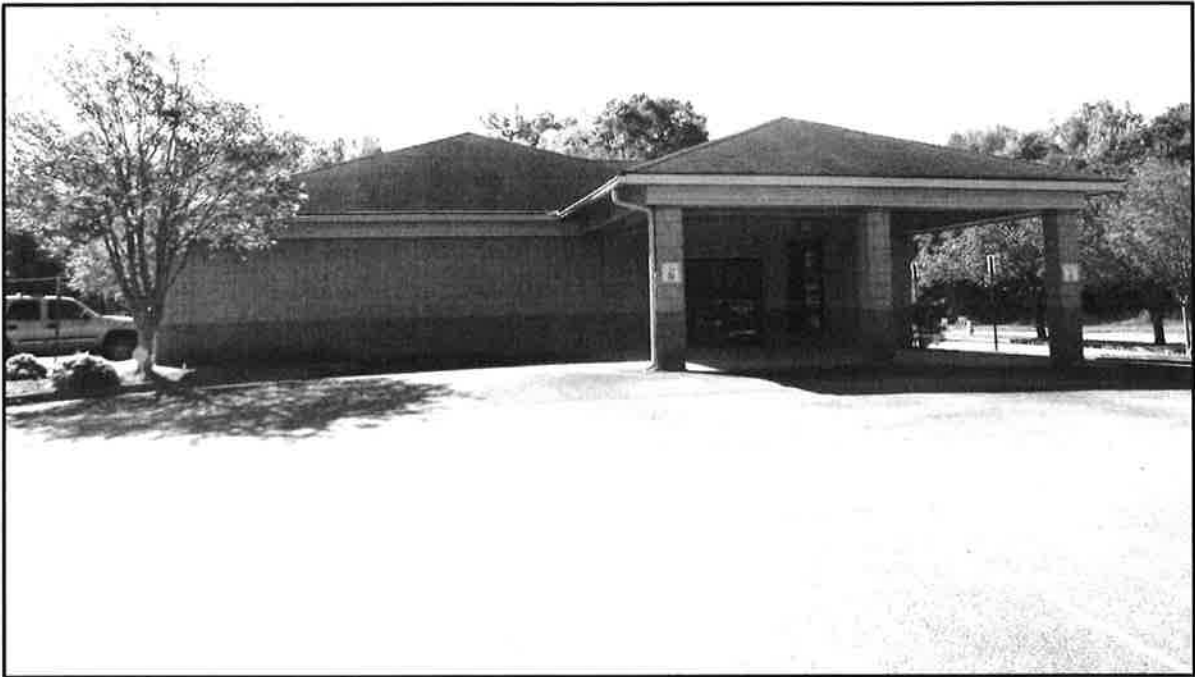
View of North Side of Subject Building
