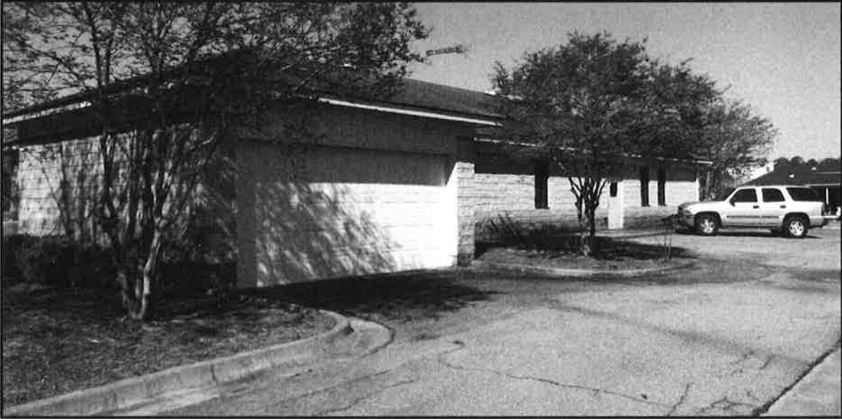
Rear View of Subject Building
